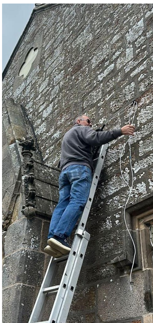
PM Donnie Mathieson installing security lights
